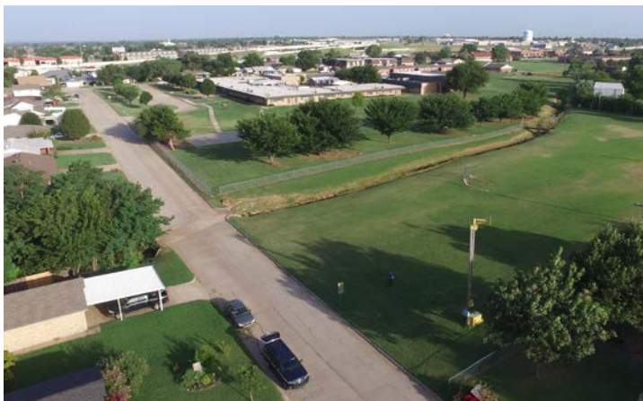
Tornado Siren #23, which protects Northmoore Elementary School and the surrounding neighborhoods. This siren has been damaged in at least two tornado events but still stands today
