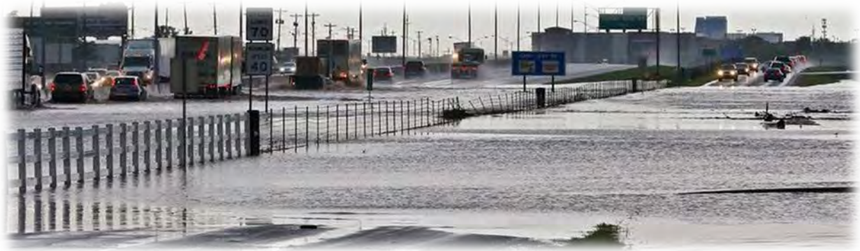
Figure 1-1: Flooding on Interstate-35 at Little River Crossing in May 2015
