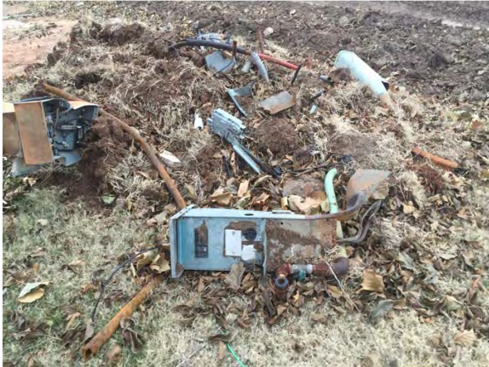
Photo 17: View of trailer infrastructure rubble from McClaren Street.
