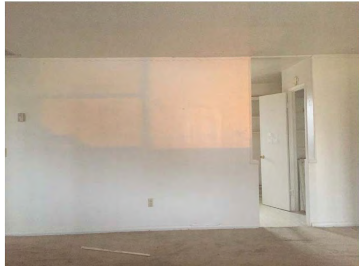
Photo 40: View of interior of 1704 McClaren Street.
