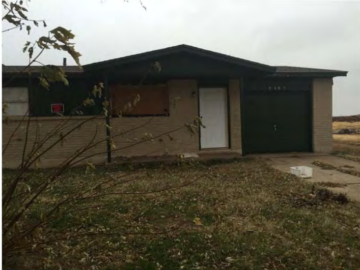
Photo 41: View of northern side of 1719 S Janeway Avenue.
