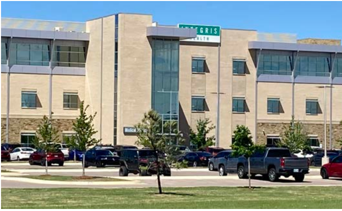
Integris Health Community Hospital at SW 34th & Telephone Rd.
