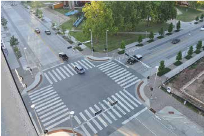
COMPLETE STREET IN OKLAHOMA CITY 180 PROJECT. THE ADDITION OF BIKE LANES, STREETScape, WIDENED SIDEWALKS AND DEFINED CROSSWALKS CREATES A SAFER ENVIRONMENT FOR PEDESTRIANS. SOURCE: A BETTER LIFE OKC BLOG, HTTP://IQC.OU.EDU/2013/11/05/BOTTOMOFTHELIST/
