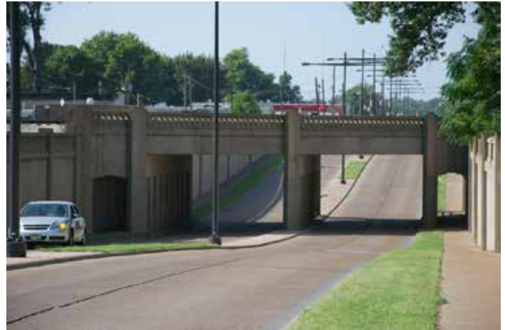
RAILROAD SEPARATED CROSSING KEEPS TRAFFIC FLOWING UNINTERRUPTED BY PASSING TRAINS. SIDEWALKS ALONG THE ROADWAY AT THESE CROSSINGS INCREASES PEDESTRIANS' AND BICYCLIST'S SAFETY AND COMFORT LEVELS. SOURCE: HTTPS://MISSPRESERVATION.FILES.WORDPRESS.COM/2014/08/UNDERPASS-AND-PEDESTRIAN-WALKWAYS.JPG
