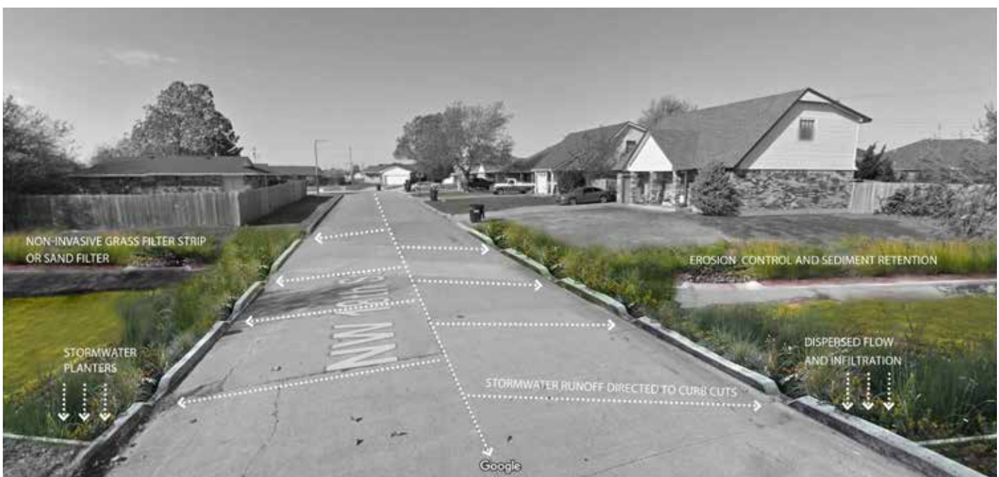
FIGURE 4.8: THE ADDITION OF STORM-WATER PLANTERS AND OTHER LOW IMPACT DEVELOPMENT (LID) TECHNIQUES OR GREEN STORM-WATER INFRASTRUCTURE (GSI) PROJECTS CAN HELP WITH STORM-WATER RUNOFF ISSUES. THESE TYPES OF PROJECTS HAVE ALSO BEEN SHOWN TO REDUCE CRIME IN THE VICINITY OF THE BEAUTIFICATION PROJECT.
